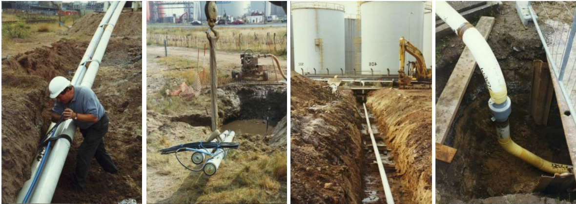
Construction Images of 6" exports in various locations in Seal Sands
